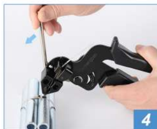
4 When the strap is tightened the left hand pulls up the cutter to cut it off, and the strap is cut off and moved away from the tie gun, so that a stainless steel band is installed
